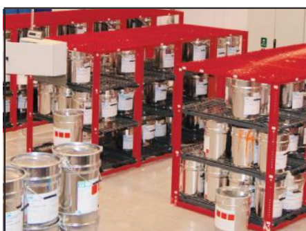
Paint store with mesh shelves to allow sprinkler water through in case of fire
